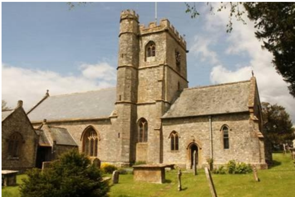
St. Stephen's receives a grant of £76,300 for the Roof Repair Fund.
